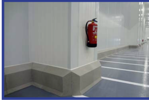
PolySto IP40F Natural installed on epoxy floor
