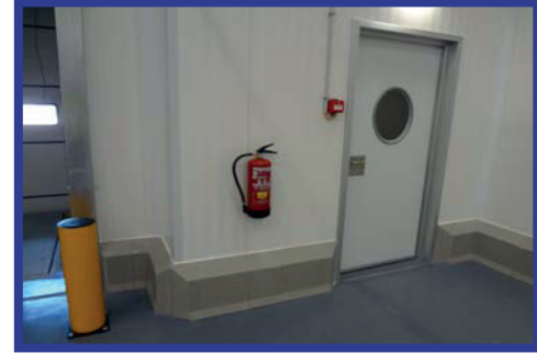
PolySto IP40F Natural installed on epoxy floor
